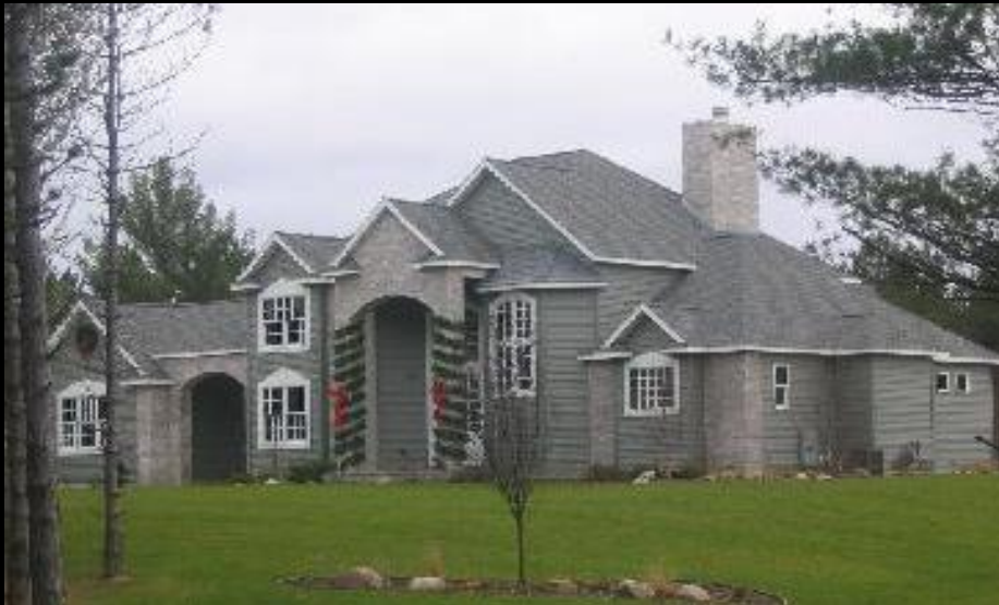
Residential and Commercial Roofing
